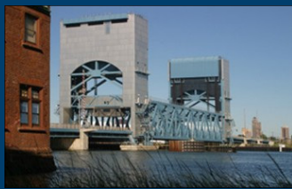
Tomlinson Bridge New Haven, CT
