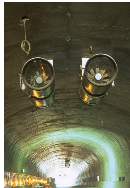
Figure 3-4. Illustration of Jet Fan Installation in a Tunnel
