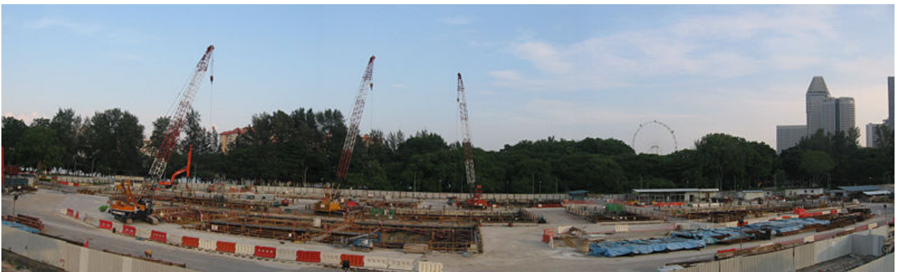
Construction site of the Nicoll Highway MRT Station.
