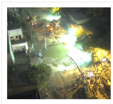
Slurry filled sinkhole
