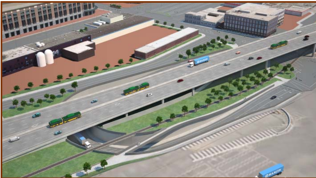
Looking east at the planned S. Atlantic Street undercrossing. The new undercrossing will ease congestion by allowing freight and other traffic to bypass train traffic.
