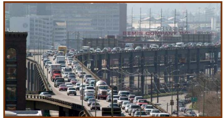
The Alaskan Way Viaduct has stood along Seattle's waterfront since the 1950s. The two-mile long structure is earthquake-damaged and must be replaced.
