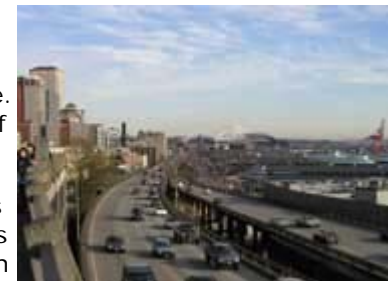
Looking south onto the Alaskan Way Viaduct.
