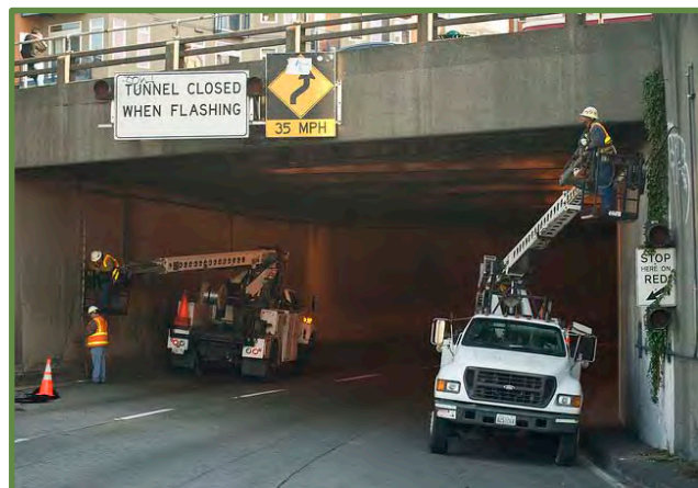
Figure 17: Battery Street Tunnel
