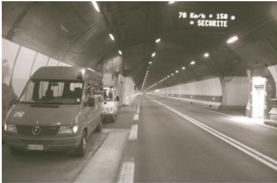
Figure 19: Emergency pullout area across from refuge room in the Mont Blanc Tunnel.
