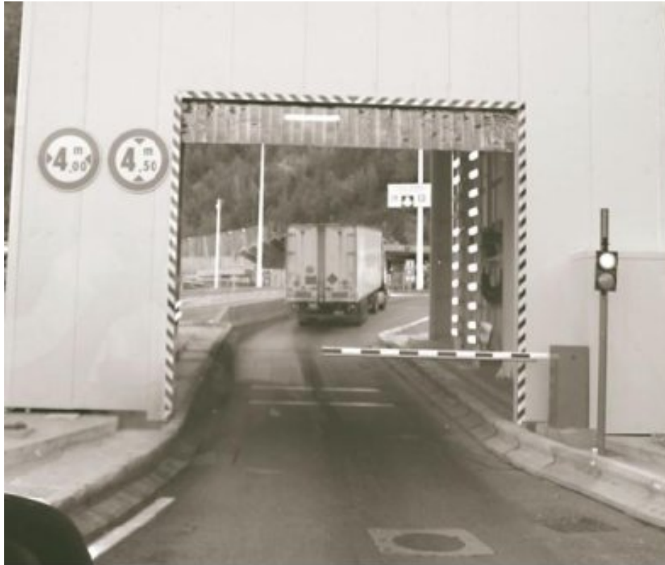
Figure 17: Truck thermal detector at the Mont Blanc Tunnel entrance.
