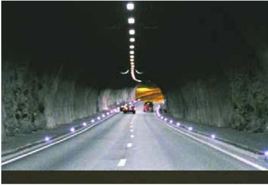
Figure 15: LED lights in the Mont Blanc Tunnel: yellow for edge delineation and blue for vehicle spacing.
