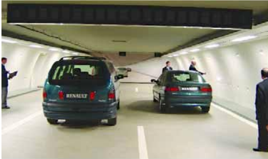
Figure 9: German end-of-queue warning vehicles Model of A86 twin roadway tube: full-size model of one section and scale model of twin tube.
