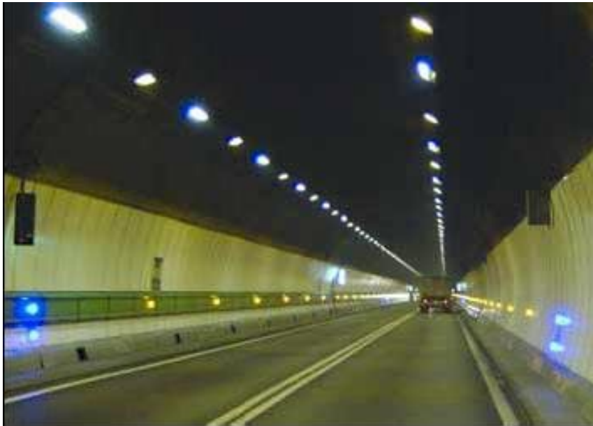
Figure 15: LED lights in the Mont Blanc Tunnel: yellow for edge delineation and blue for vehicle spacing.
