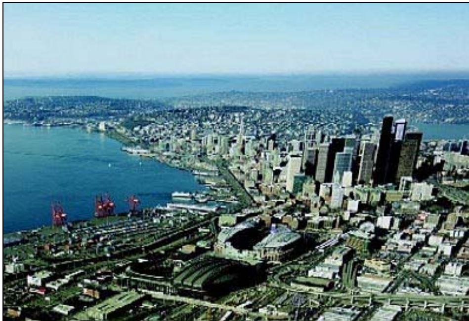
13 Figure 3-1. Aerial view of Alaskan Way Viaduct along Stadiums and 14 Waterfront
