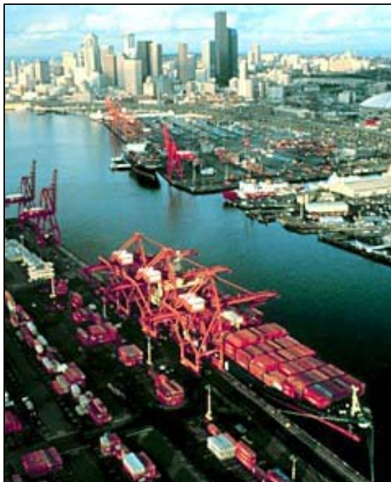
20 Figure 4-1. Urbanized Shoreline of Duwamish River East Waterway and 21 Coast Guard Vessel Slip (lower right of photo)
