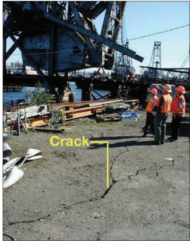
Figure 4-13. Piers on BNSF Railway West Seattle bascule bridge moved together 6 inches in the Nisqually earthquake due to movement of the soil behind the abutment toward the water, then several inches more in the next few days.
