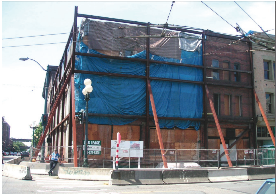
Figure 5-2: Unreinforced masonry building damage, 2001 Nisqually earthquake.
