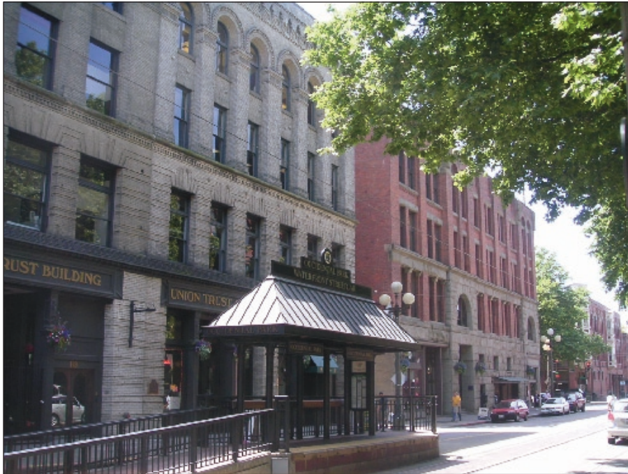
Figure 7-3: Pioneer Square. Late 19th and early 20th century construction (some of it retrofitted) on liquefiable soil.
