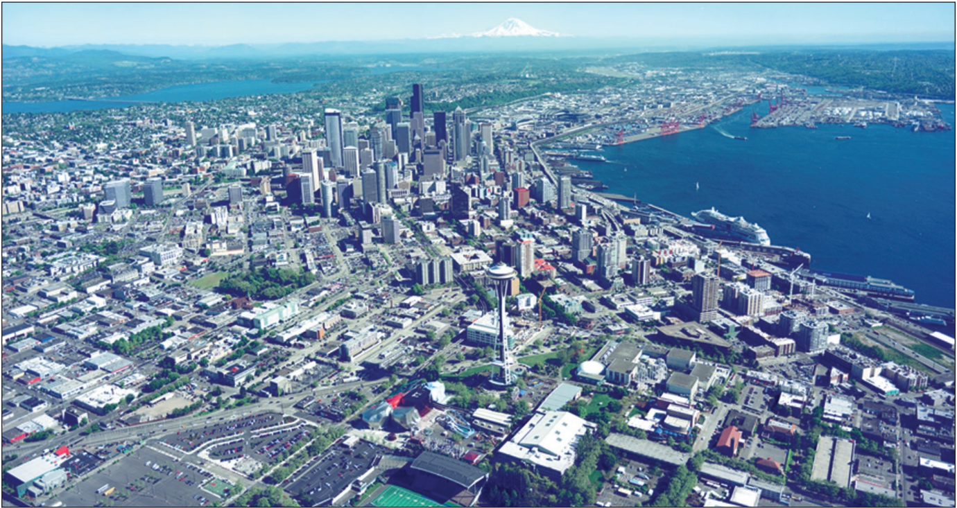
Figure E-3: Repair of damaged transportation systems will be the most critical economic restoration initiative facing the Central Puget Sound region after the scenario Seattle Fault earthquake. The quicker transportation systems are repaired, the quicker the region will recover from the earthquake.
