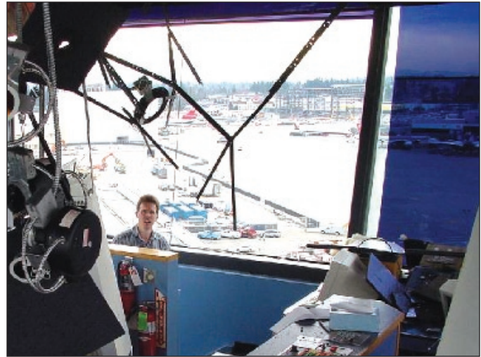
Figure 4-8: Nonstructural damage in the old Sea-Tac International Airport control tower from the Nisqually earthquake.
