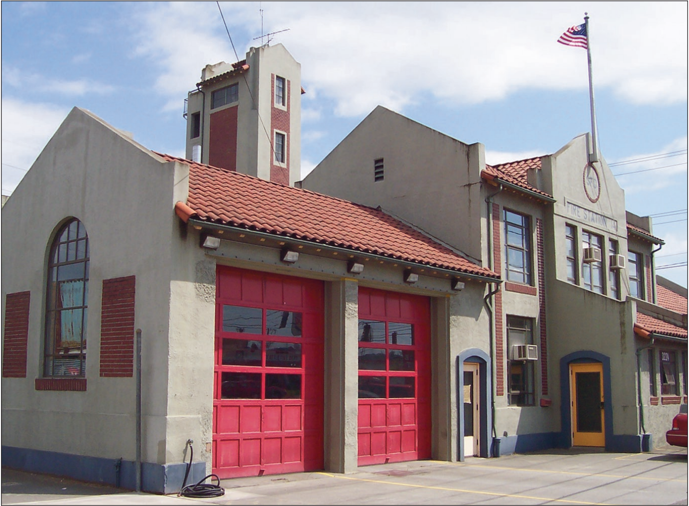
Figure 6-5: A typical Seattle fire department station. Note the hose tower and wide apparatus doors.
