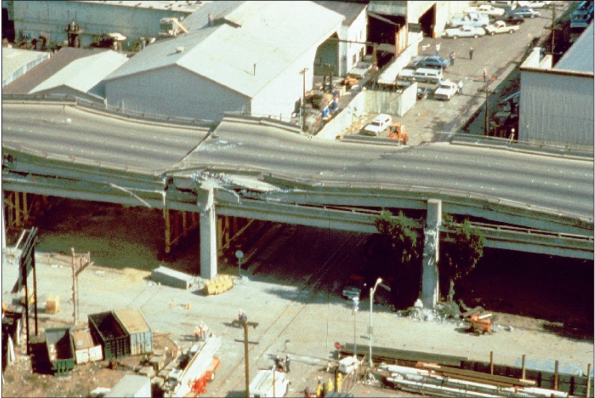
Figure 8-3: Damage to transportation routes will make it difficult for commuters in the Central Puget Sound region to return home following the scenario M6.7 earthquake. The Alaskan Way Viaduct, which carries one-quarter of all traffic through Seattle, is similar in age and construction to the Cypress Structure of the Nimitz Freeway in Oakland (above), which collapsed during the 1989 M6.7 Loma Prieta earthquake.
