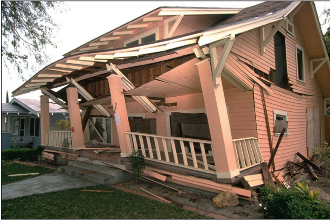
Figure 8-8. Damage to single-family homes and other residential structures will temporarily displace about 46,000 households after the scenario Seattle Fault earthquake. Among the damage that will be seen is unreinforced, poorly bolted or unbolted homes being shaken off their foundations. Photo / Federal Emergency Management Agency
