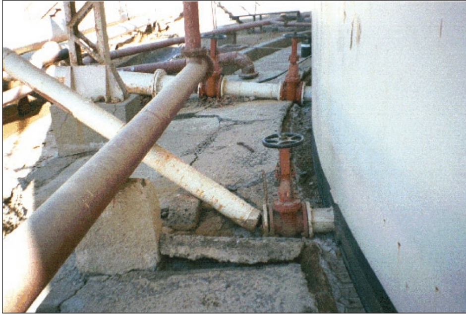
Figure 5-15: Fuel storage tank base settlement, 300mm sliding and broken pipes.
