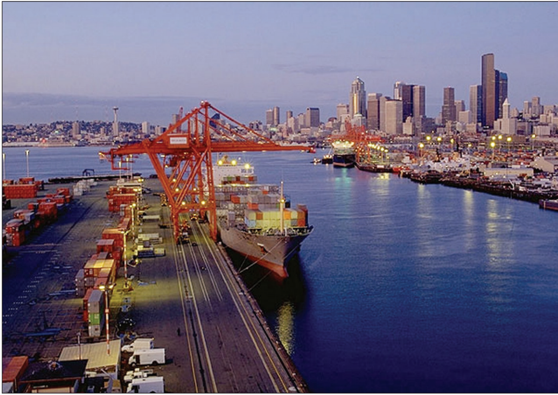
Figure 4-10. The Port of Seattle. Photos / Don Wilson, Port of Seattle
