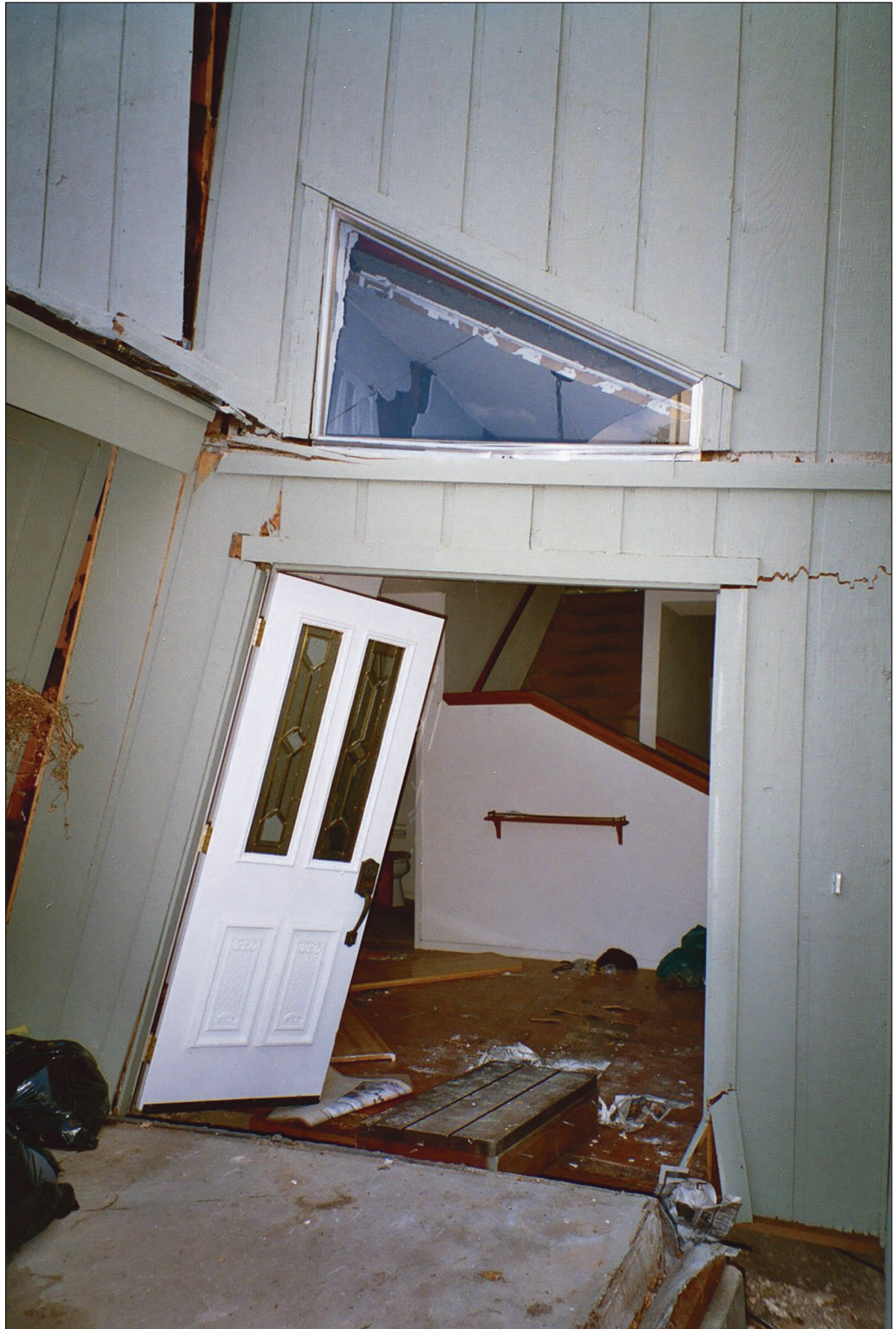
San Simeon, CA earthquake 2003. Photo / Federal Emergency Management Agency
