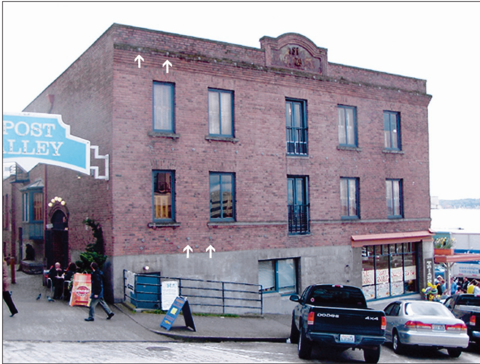
Figure 5-3: Undamaged retrofitted unreinforced masonry building in Seattle. Note bolts in side of building where anchors have been placed (see arrows).
