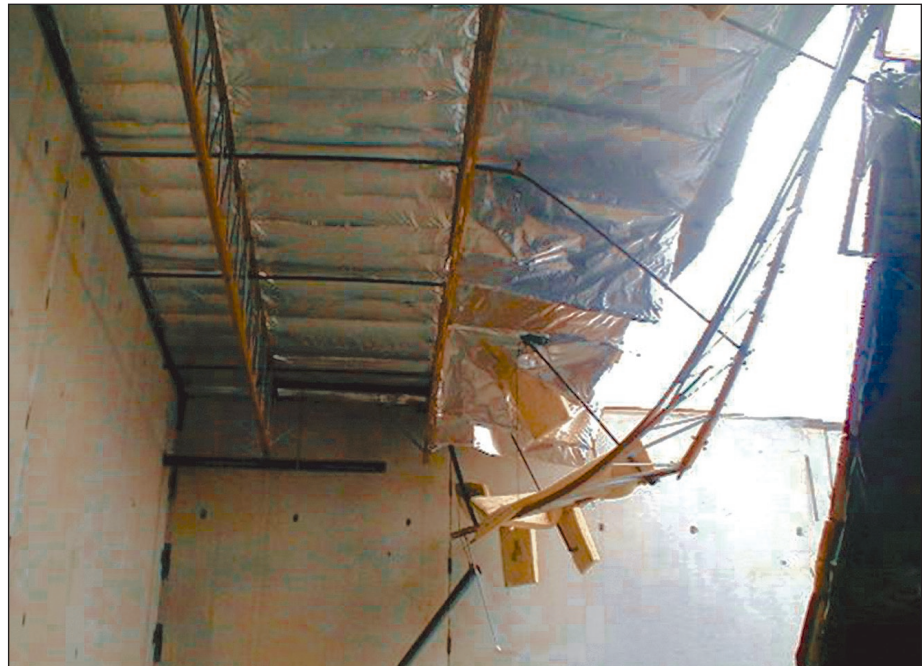
Figure 5-5: Tilt-up building damage, 2001 Nisqually earthquake.
