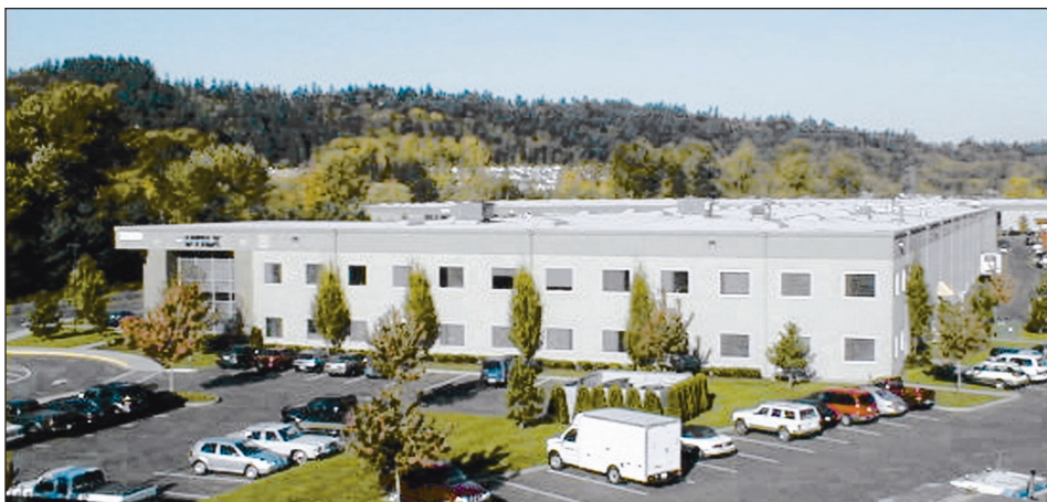
Figure 5-4: Example tilt-up building in Seattle.
