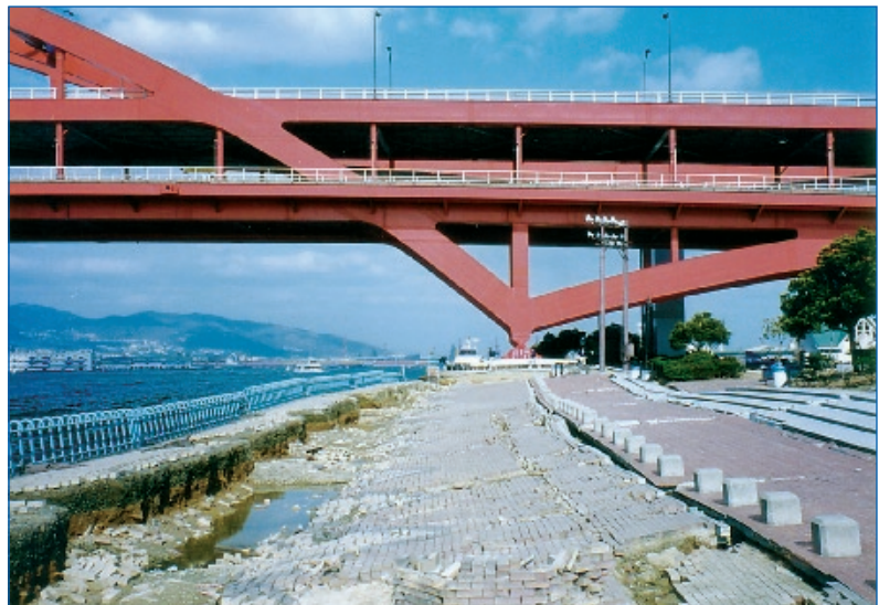
Figure 2-4: Damage from lateral spreading at Port Island Bridge during the 1995 M6.9 Kobe earthquake. Similar and more significant damage is expected during the Seattle Fault scenario earthquake.
