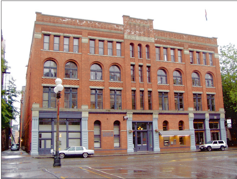
Figure 5-1: A representative unreinforced masonry building in Seattle.
