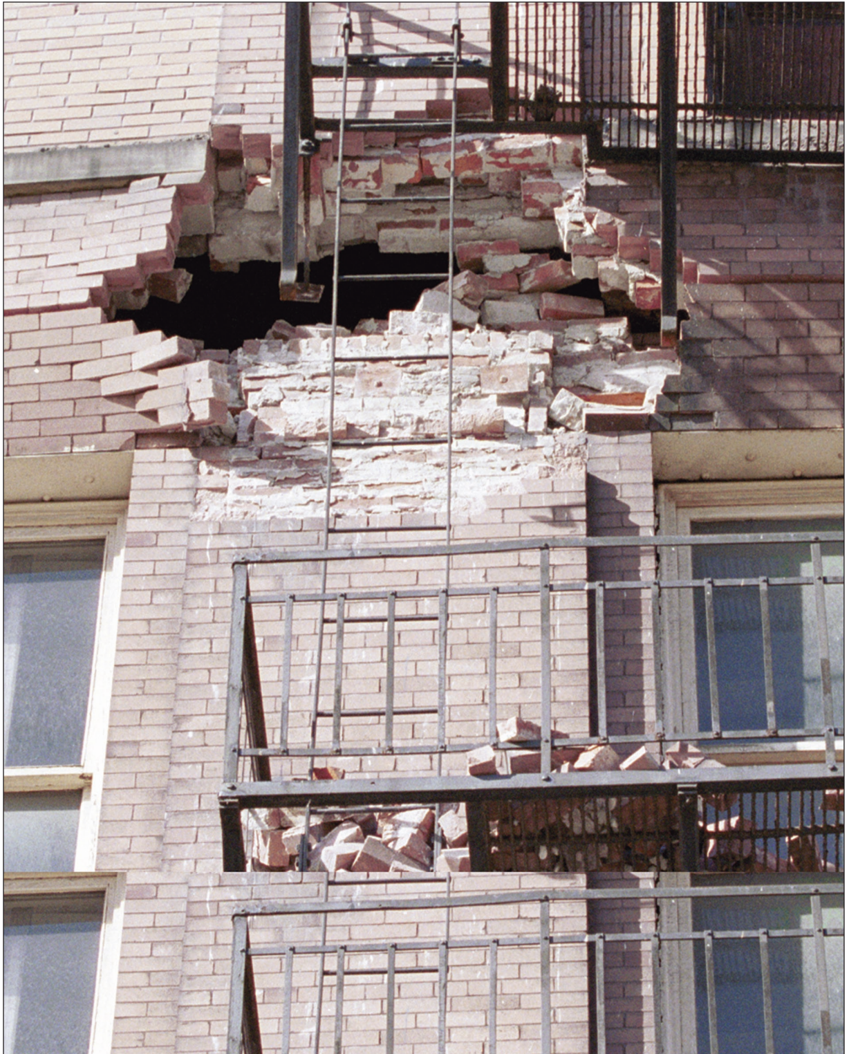
Nisqually earthquake 2001. Photo / Federal Emergency Management Agency
