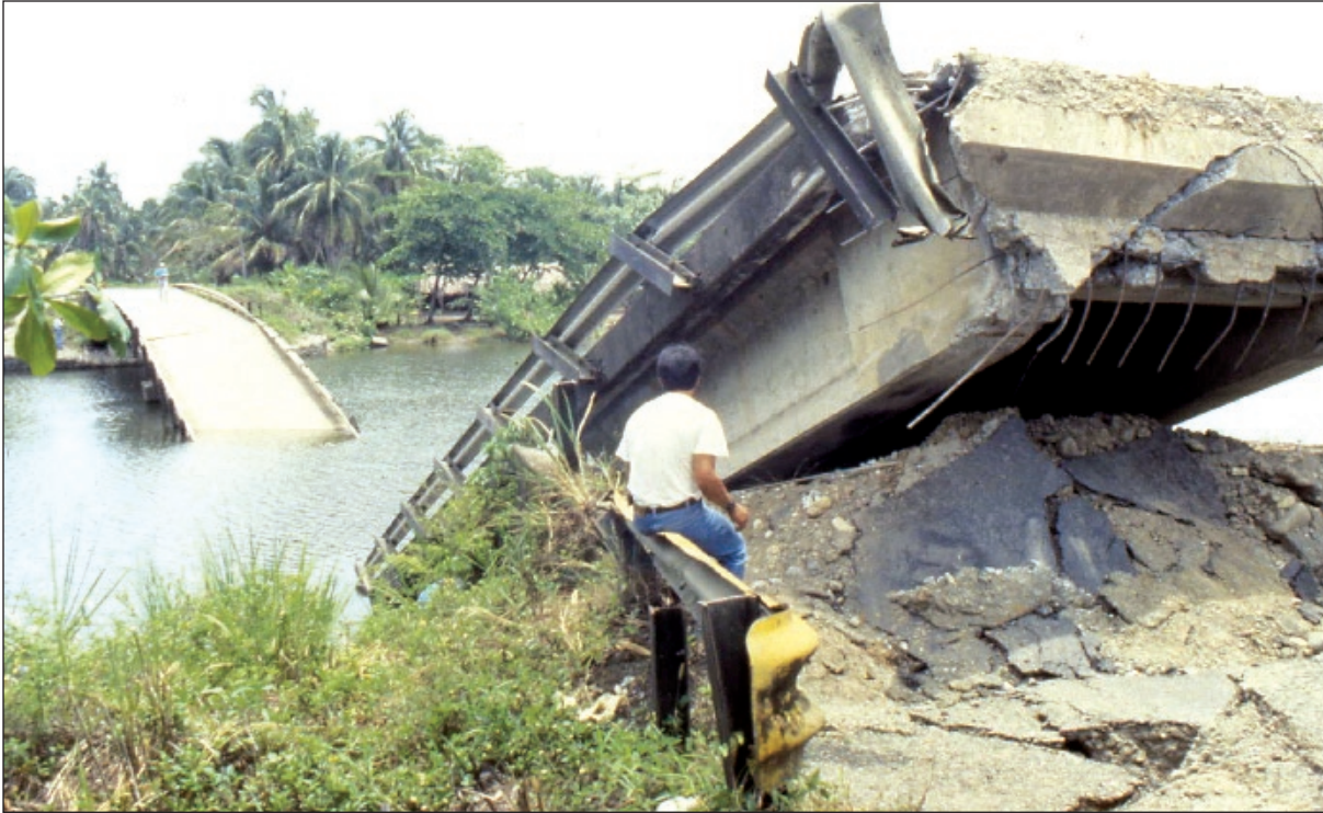
Figure 4-5: Bridge damage from the 1992 Costa Rica earthquake.
