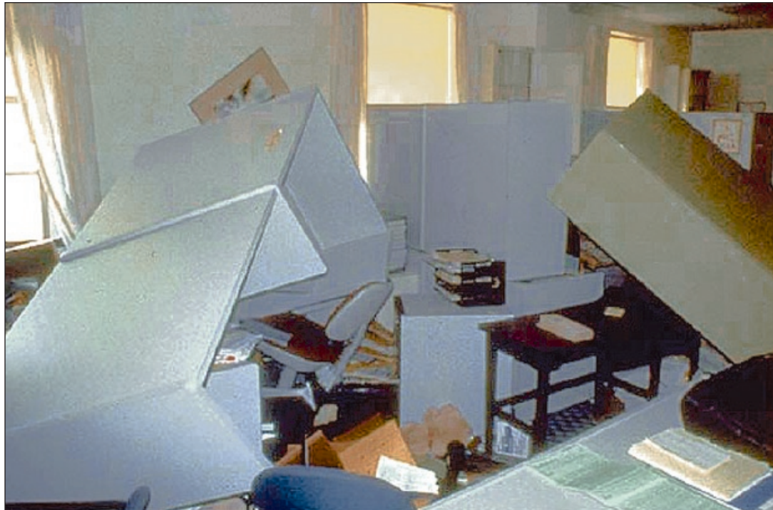
Figure 6-3: Typical nonstructural damage.
