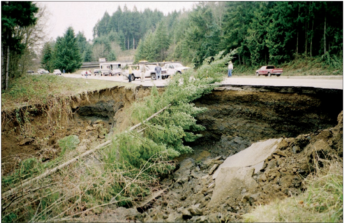
Figure 4-7: Highway 101 damage from ground failure caused by the Nisqually earthquake.
