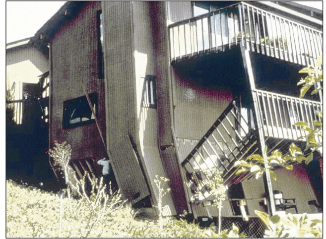
Figure 5-11: Strong ground shaking can damage multi-story buildings in the same way it can damage single-family homes. This apartment building slid off its foundation because it was not bolted or had been poorly bolted to its foundation. Photo / Applied Technology Council
