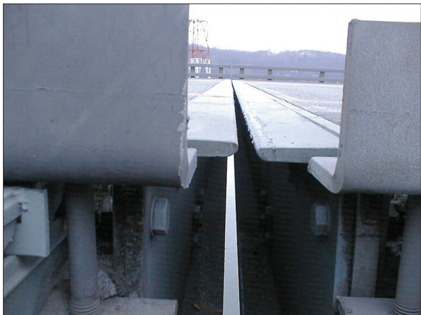
Figure 4-6: Moveable bridge alignment problems after Nisqually earthquake.
