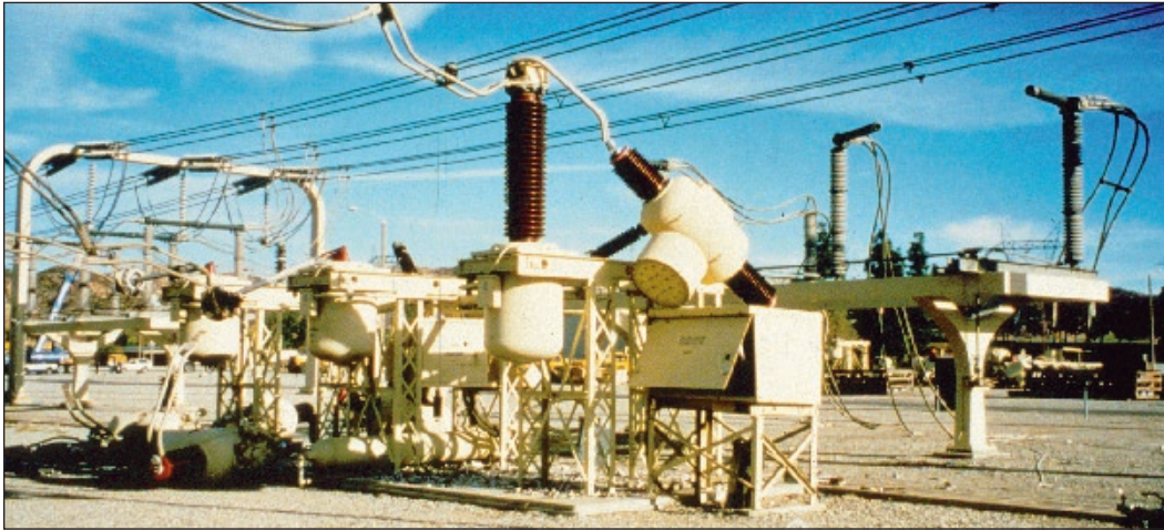
Figure 3-6: Electrical substation damaged by 1994 Northridge earthquake. Similar damage will occur in a major Seattle Fault earthquake.
