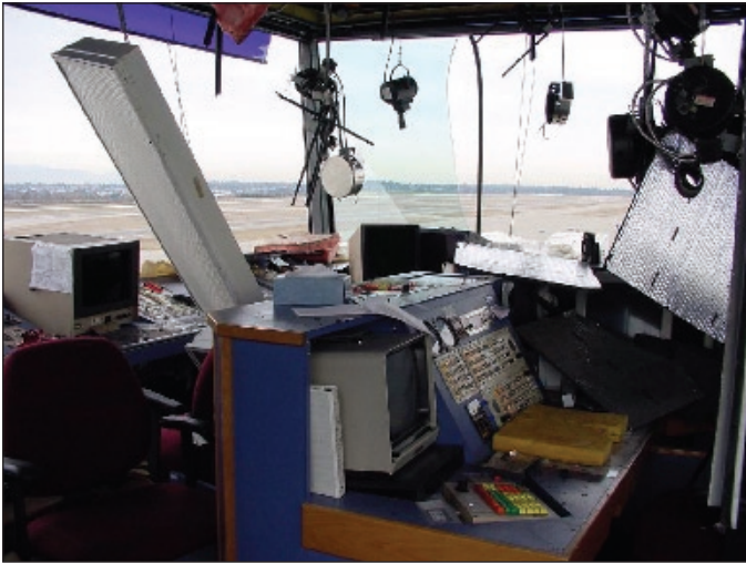
Figure 4-8: Nonstructural damage in the old Sea-Tac International Airport control tower from the Nisqually earthquake.
