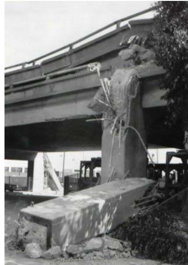
Cypress Viaduct (Loma Prieta, 1989)
