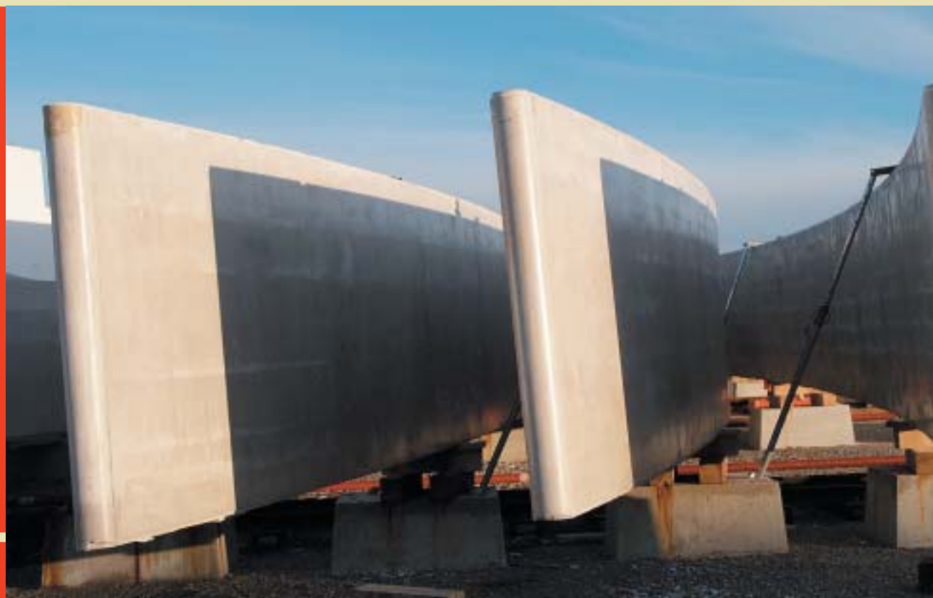
Voussoirs: impressive dimensions for the toll barrier canopy.
