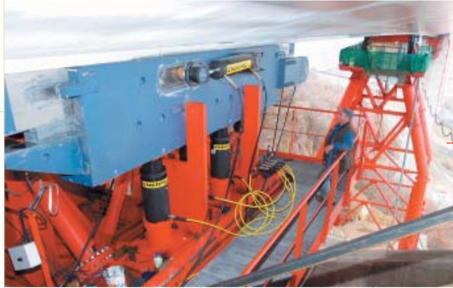
It is with the help of transfer jacks that the thousands of tons of the deck can be lifted and moved forwards.
