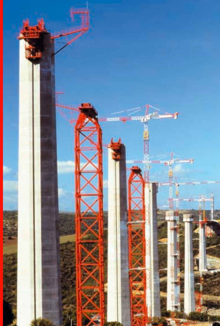
Seven concrete needles, erected on time
