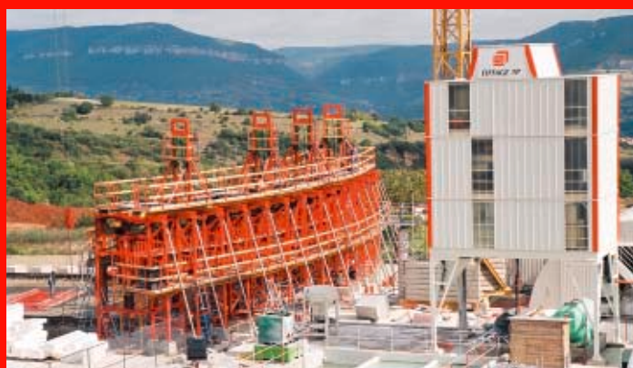
Construction of the canopy for the toll barrier: a twisted "leaf" of concrete, 100 metres long and weighing close to 2,500 tons.
