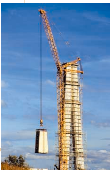
Raising a temporary pylon to relieve the strain on the deck's leading edge.
