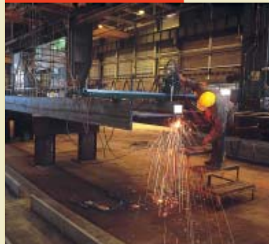
A goldsmith's precision for assembling the box girder sections.
